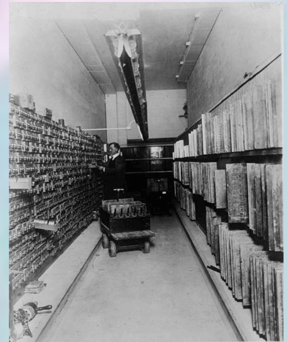
Interior of plate and die vault at the BEP left: roll case; right: engraved plates
